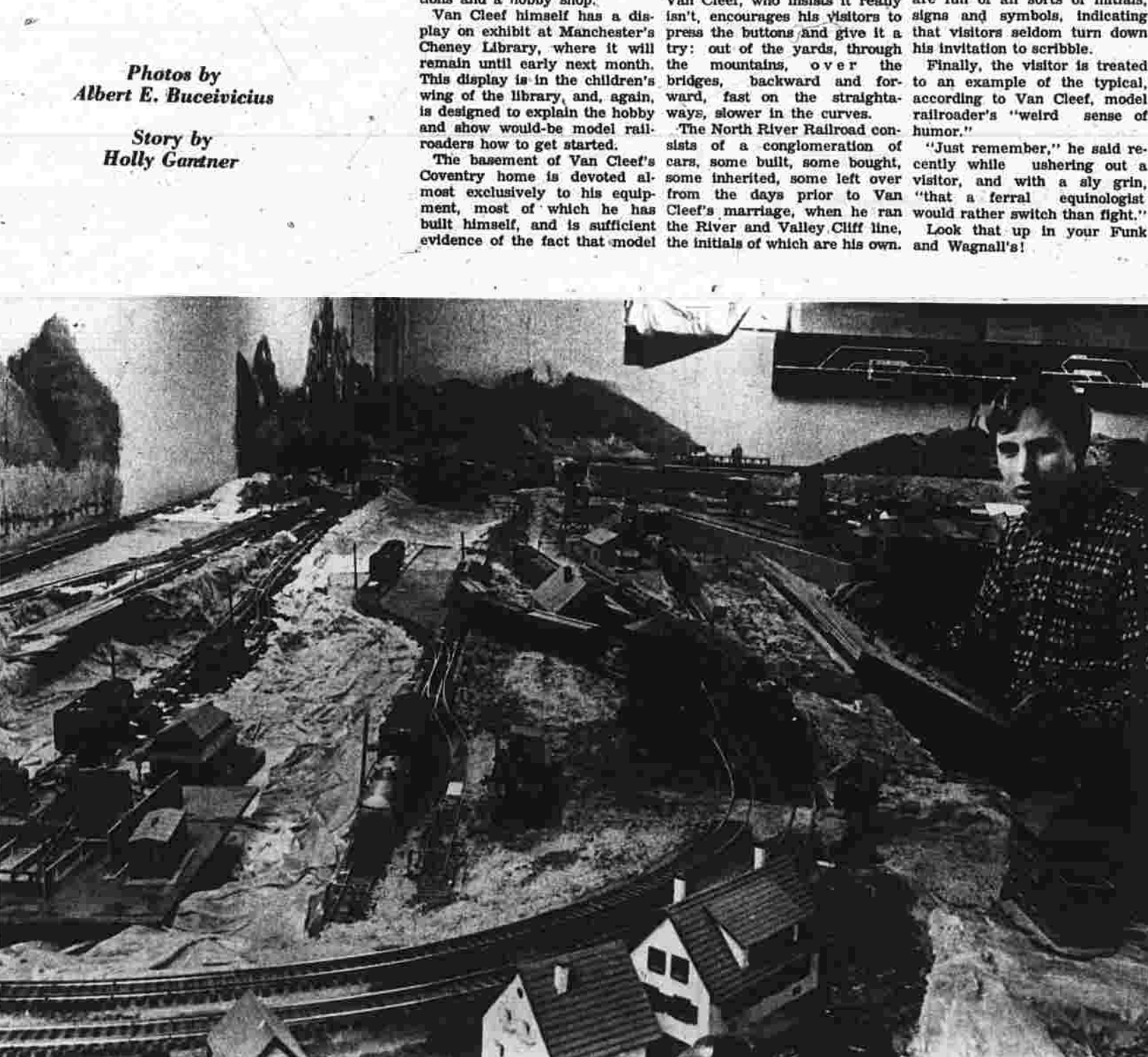
Engineer VanCleaf guides '99 into town right on schedule.
