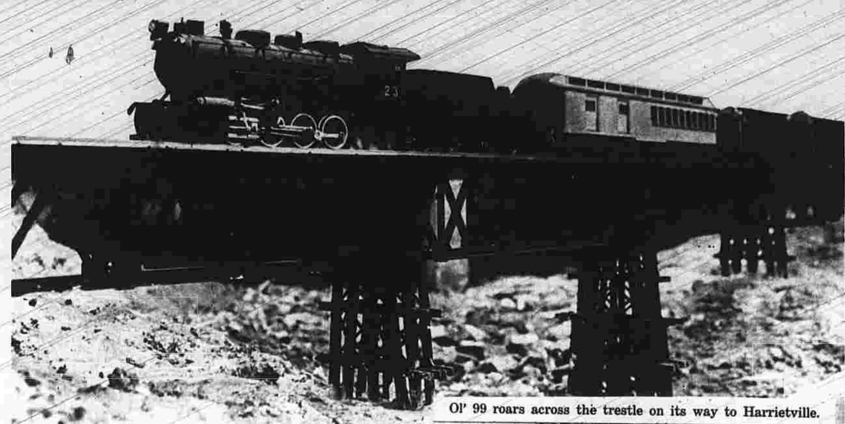
Of 99 roars across the trestle on its way to Harrietville.
